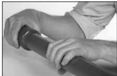
After completing the joint it must be held together for a brief time while the cement begins to dry. This is to prevent the pipe from squirting back out of the fitting socket. The phenomena occurs because fresh cement is an excellent lubricant and product standards dictate the socket to be
