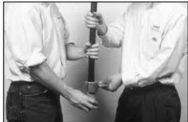
3. Simultaneously, installer #1 should place the pipe and installer #2 should place the socket connection squarely on the Heating Anvils (heat face sets) so that the ID of the connection and the OD of the pipe are in contact with the heating surfaces. Care should be taken to insure that neither the pipe or socket connection are
