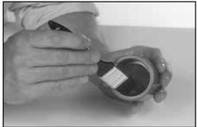
6. Put a second coat of solvent cement on the pipe-end. This completes the six steps of alternate surface application for a joint – three of primer and three of cement – starting with the female component. Cement layers on the pipe must be without voids and sufficient to provide an immediate and continuous wet filet around the socket entrance radius/
